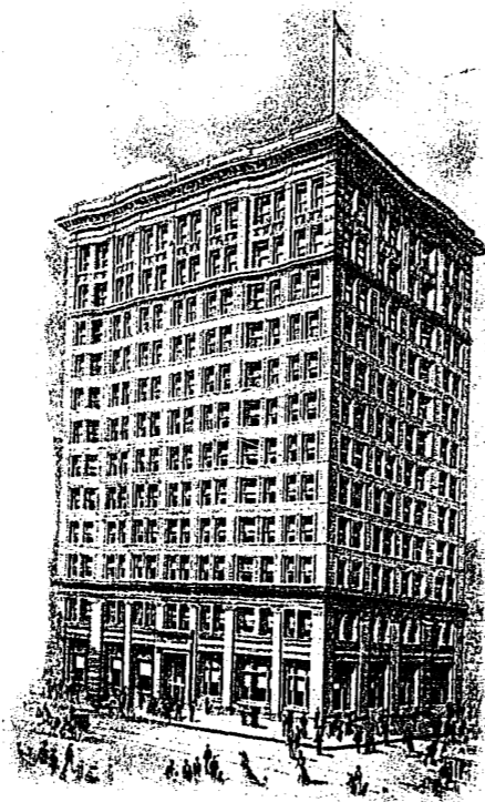
HIBERNIA BANK BUILDING, NEW ORLEANS, LA.
